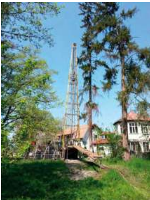
Figure 14. Aspects from the execution of the AHR piezometer in April 2015
